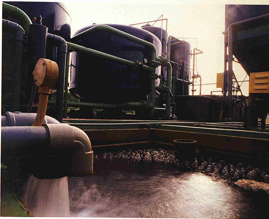
Water treatment in a modern factory in Selangor. Responsibility is the keyword in modern industrial management. Factories have to avoid polluting the environment and harming the world that we live in.
