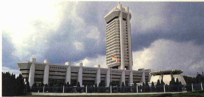
The State Secretariat building in Shah Alam. This is the seat of the Selangor government.
