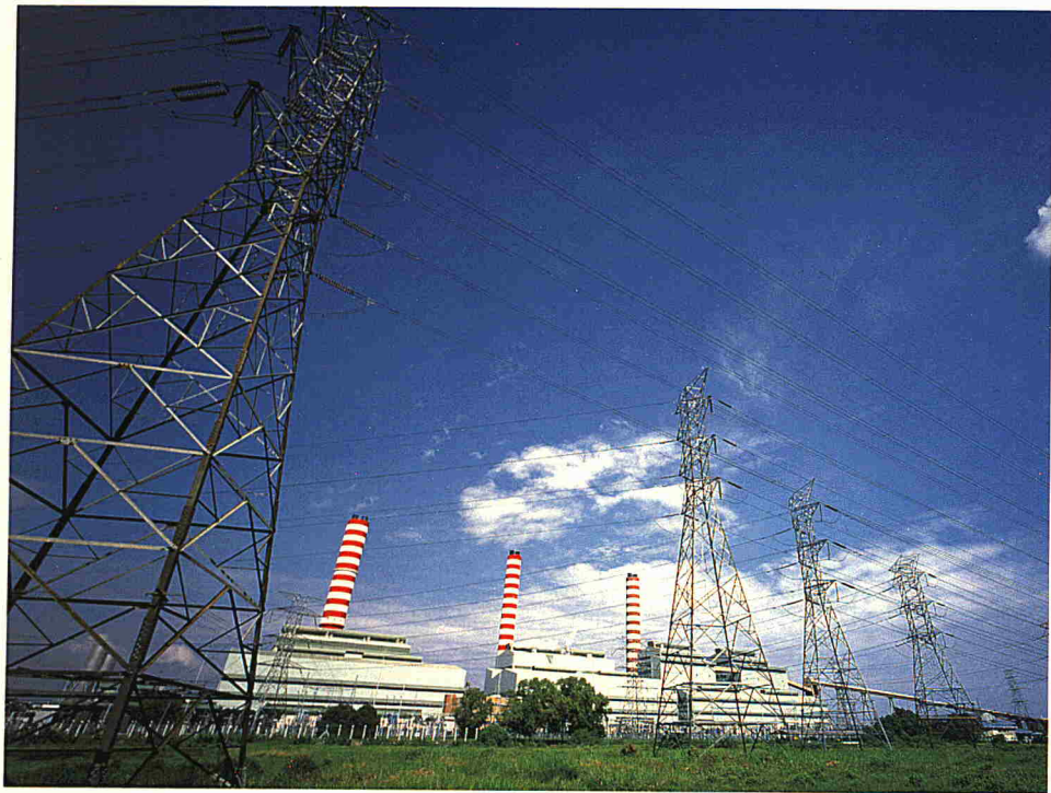
Energising the nation, meeting the needs of domestic and industrial users. Power pylons rise over the landscape in urban and rural areas. Meeting the energy needs is one of the priorities of state planners. This power station is in Kapar, Klang. Energy demand is expected to surge in 2005 when Selangor becomes fully industrialised.
